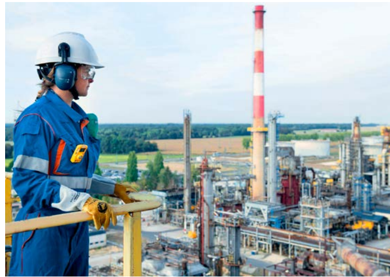
Operator at the Grandpuits zero crude platform.
