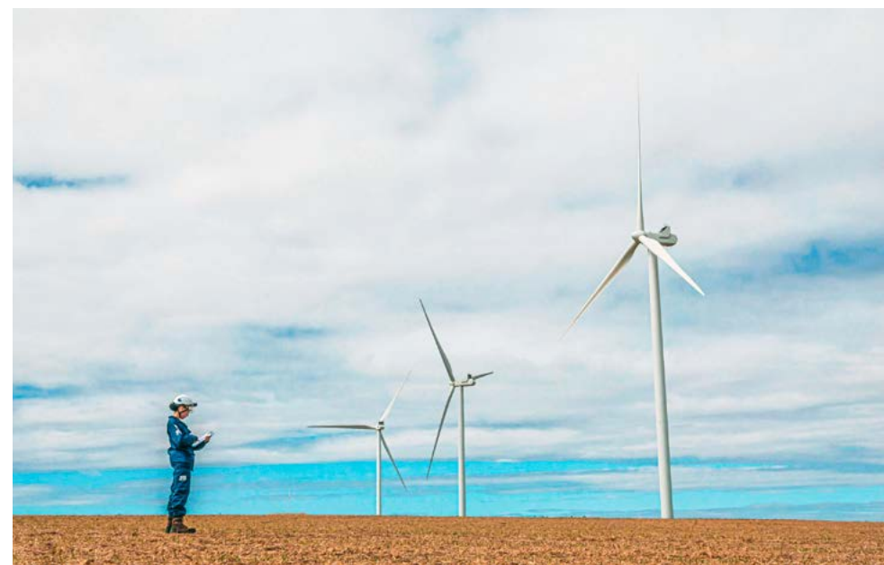
Maintenance operations on the Champagne Conlinoise wind farm (France).
