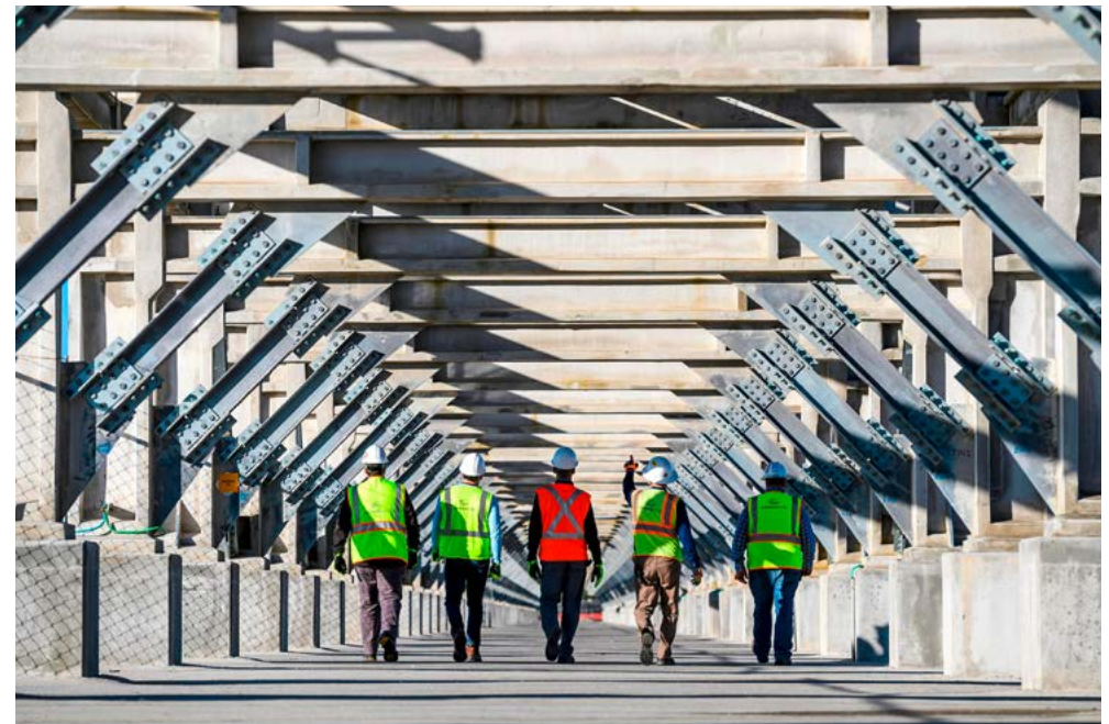
Liquefaction terminal (US).
