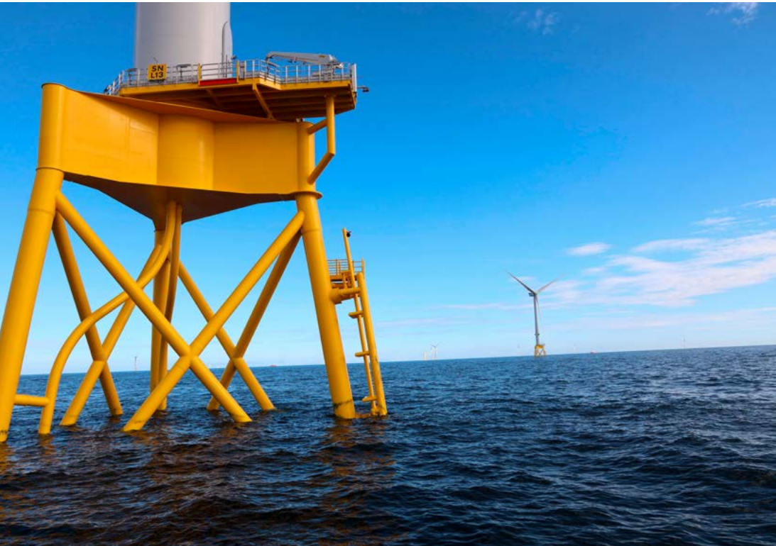
Seagreen (Scotland) offshore wind farm under construction.
