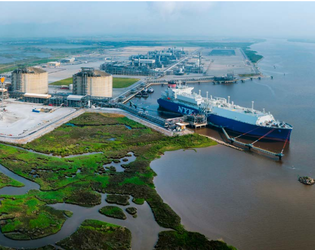
First loading of the LNG Adventure vessel at the Cameron LNG liquefaction terminal in Louisiana (US).
